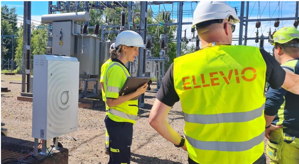
Currently, the project has been focused to the measurement and monitoring of SF<sub>6</sub> gas at one of Ellevio's substations in central Sweden. However, by connecting more sensors to the SIPP Hub, the solution can be used in virtually all areas. The data gathered will provide network owners with an immediate insight into the need for maintenance, while also detailing other factors that could impact on operational reliability.
